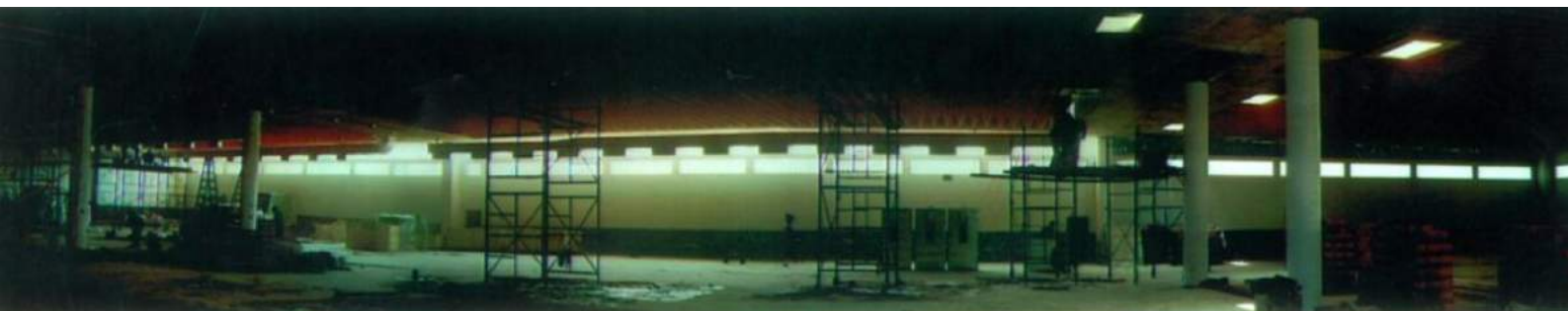
Industrial building in 1987 with a 100x70m structured supported only on 4 interior columns and the perimeter.
