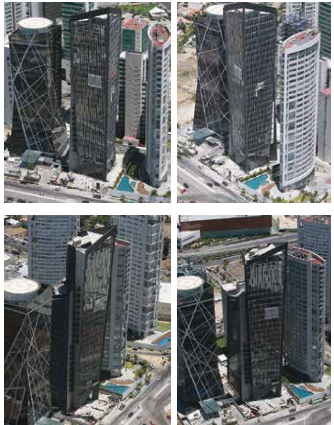
Fig. 1: The Cube II is an office tower with 29 above-ground levels and seven underground parking levels. The office levels are configured as two modules (wings) tied to common core containing the vertical circulation. Each of the two office wings has a triangular shape with the column at the apex inclined at 4 degrees to the vertical
