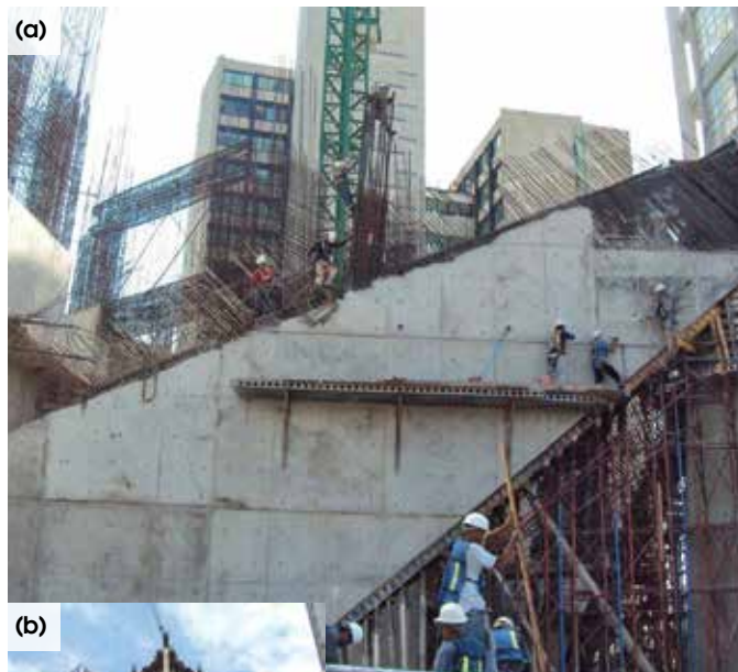
Fig. 7: The main entrance of the building (front) is framed by inclined transfer girders: (a) a transfer girder is shown during construction in July 2011, as workers are placing the reinforcing bars for the intermediate side column above; and (b) the completed girders are shown in this view, taken in February 2012
