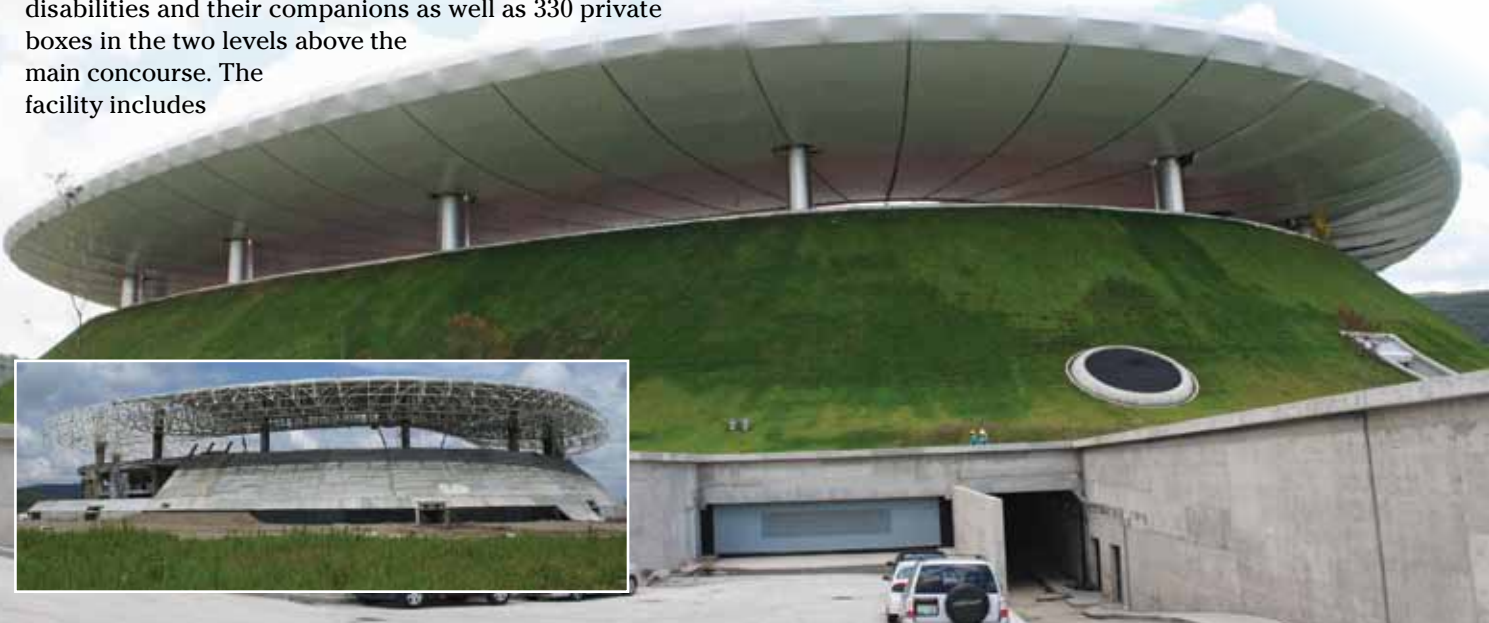
Fig. 1: Omnilife stadium in Guadalajara, Mexico. Inset: The “volcano and cloud” take shape. Access to the stadium is gained through a large opening through the volcano. The large opening (shown in the inset) and five smaller openings provide egress. The volcano is formed by a truncated cone formed of concrete. This feature significantly reduces potential seismic loading and provides a beautiful, 20 m (65 ft) tall meeting place on the main concourse
