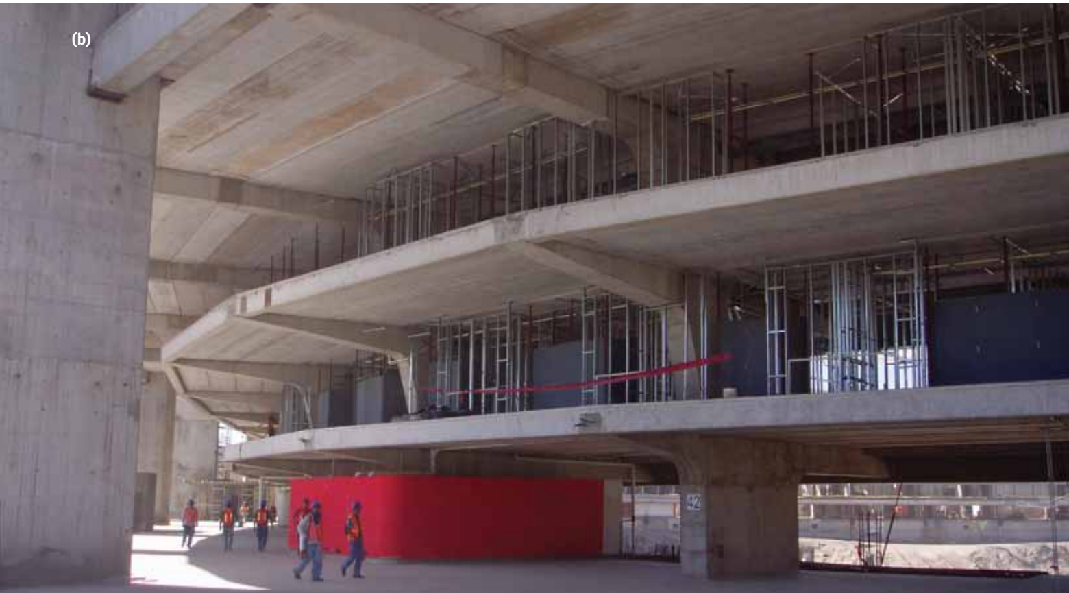
Fig. 4: The private box levels comprise field-topped precast floor elements and precast seating units supported by post-tensioned double cantilever beams: (a) in April 2008, construction of the lower level was underway; and (b) in March 2009, the structure for the two private box levels and upper concourse levels was nearly complete
