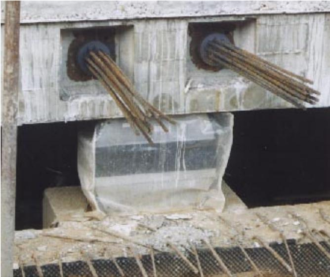
Fig. 6: Base isolation unit and post-tensioning anchorages
