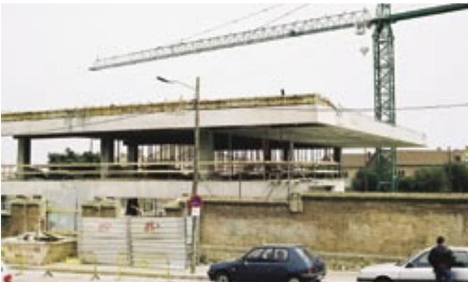
Fig. 7: Partial view of the finished structure showing a long cantilever roof at Block 1
