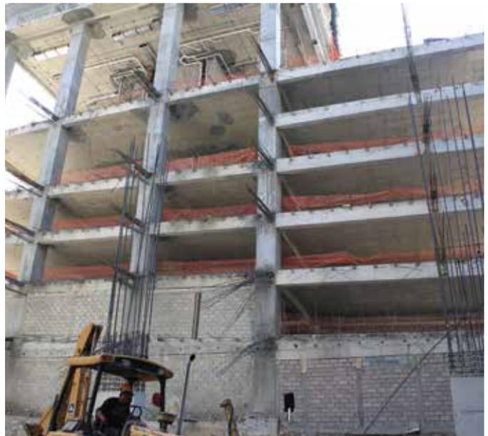
**Fig. 5: Parking zone construction. Girders and lightened PT concrete slabs are sloped**
