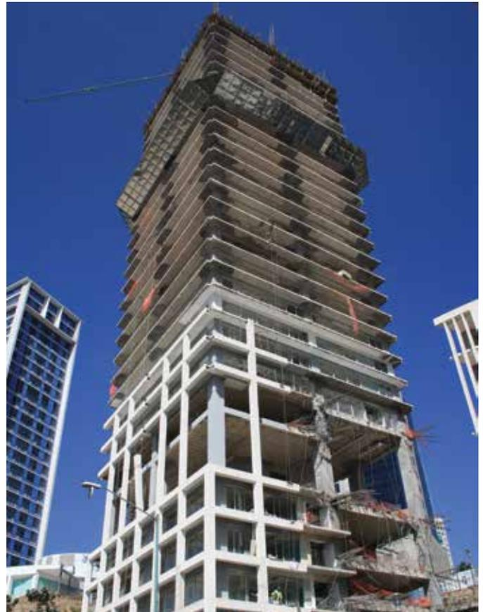
**Fig. 7: A progress photo taken in April 2013, showing the construction process for the architectural white precast façade elements**
