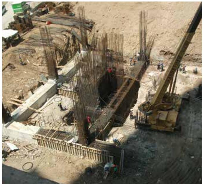
**Fig. 3:** The building was founded on 18 drilled shaft foundations, with one shaft per column and nine shafts supporting the concrete base slab at the central core
