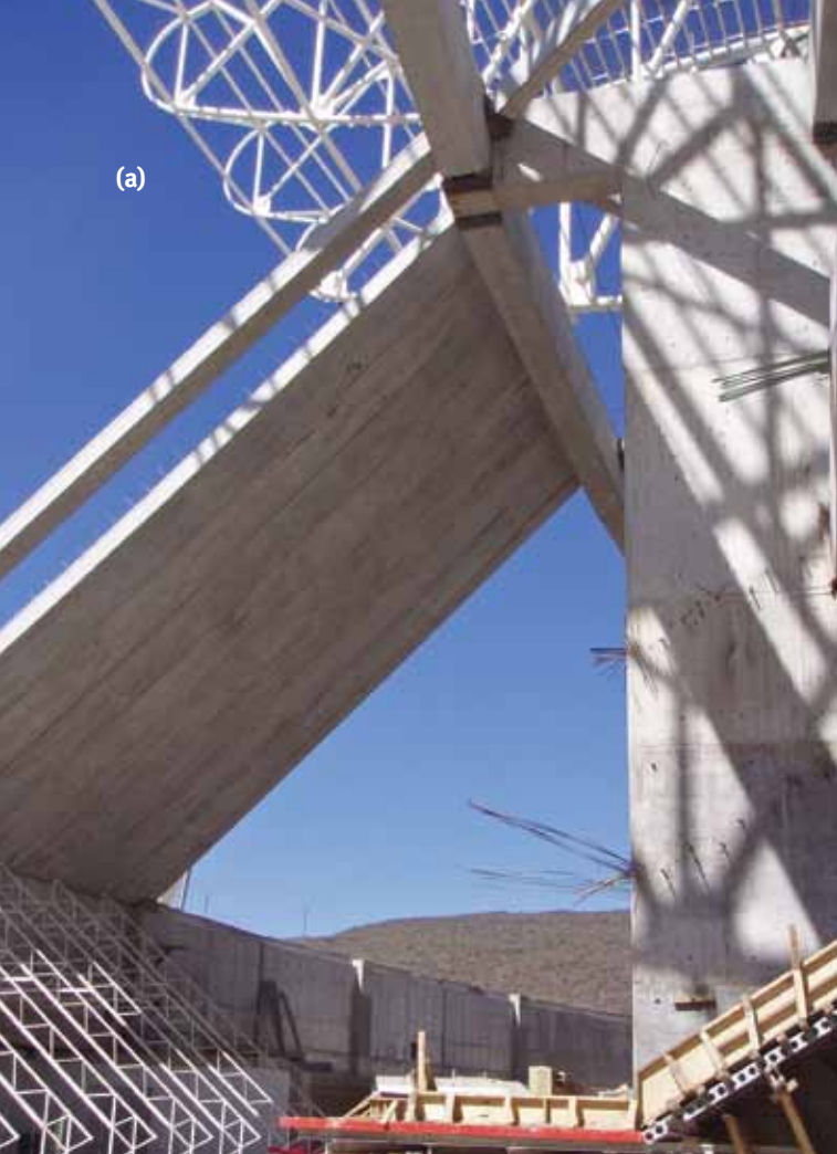
Fig. 2: Construction of the berm of the volcano. The upper support for the slab units consists of a horizontal diaphragm with two ring beams connected by diagonal struts: (a) view from the concourse as a slab unit is installed in the berm. In the foreground, stair formwork is assembled at a secondary column ( photo courtesy of Juan Pablo Beas ); and (b) view from the stairs leading to the upper concourse, showing a macrocolumn in the foreground and a secondary column (with stair formwork) in the background
