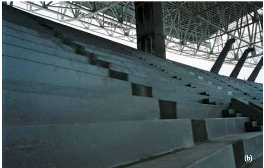
Fig. 7: Precast-prestressed seating elements were produced on site: (a) units included exposed passive reinforcement for subsequent embedment in continuity joints at raker beams; and (b) the continuity joints for the precast seating units (dark concrete) help to avoid leakage from rain and drinks, and they reduce crowd vibration issues, both common problems with simply supported seating units
