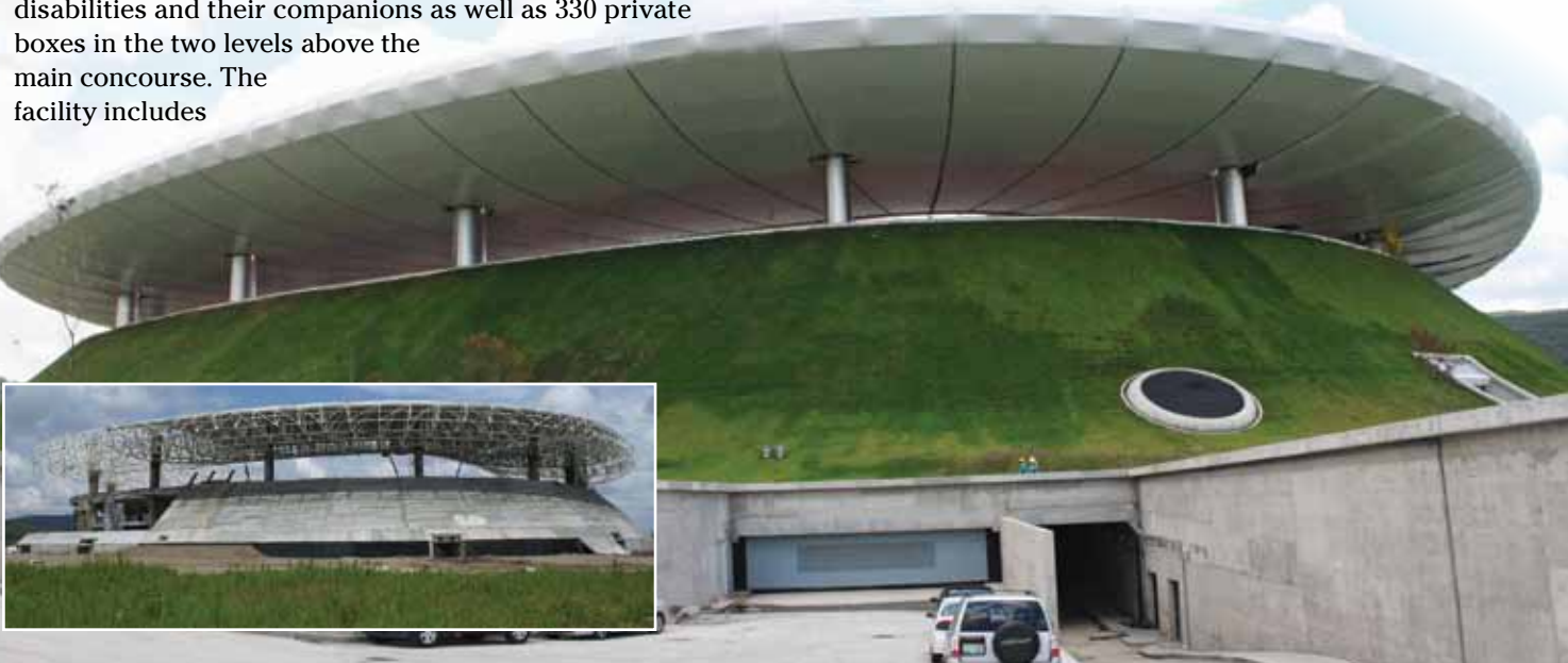
Fig. 1: Omnilife stadium in Guadalajara, Mexico. Inset: The “volcano and cloud” take shape. Access to the stadium is gained through a large opening through the volcano. The large opening (shown in the inset) and five smaller openings provide egress. The volcano is formed by a truncated cone formed of concrete. This feature significantly reduces potential seismic loading and provides a beautiful, 20 m (65 ft) tall meeting place on the main concourse
