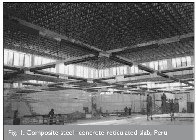
Fig. 1. Composite steel–concrete reticulated slab, Peru
