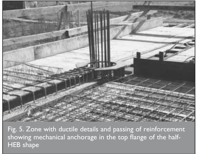
Fig. 5. Zone with ductile details and passing of reinforcement showing mechanical anchorage in the top flange of the half-HEB shape
