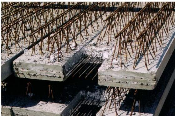
**Fig. 5: The slab blockout shown here is used in a dropped slab panel spanning between columns and allows the column vertical reinforcement to pass through the precast panel**
