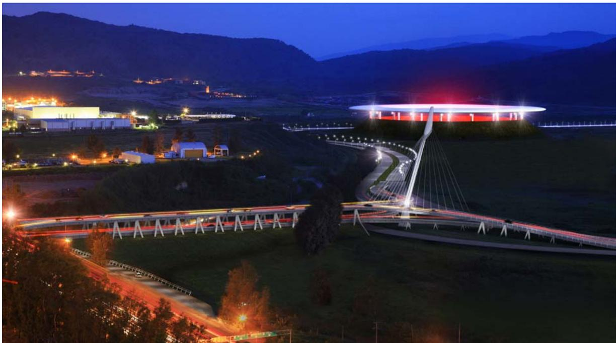
**Fig. 8: JVC overpass including a singular curved cable stay bridge shown at the center. Left and right bridges are formed by pre-stress slabs and conventional or postensioned girders, according to their span resulting in a totally 1m flat system. On the back the chivas soccer team stadium that we designed using also prestress slabs.**
