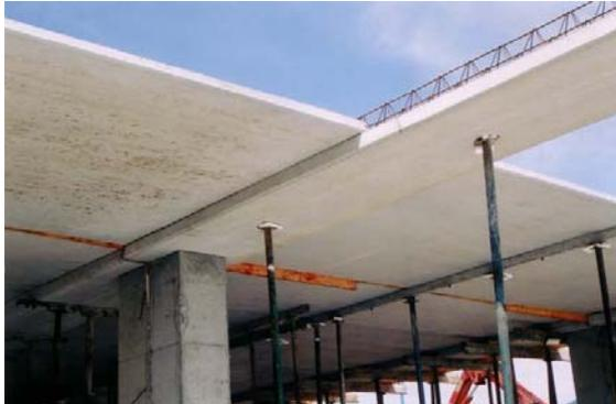
**Fig. 4: Dropped precast slabs spanning between the columns partially support the precast slabs spanning in the other direction**
