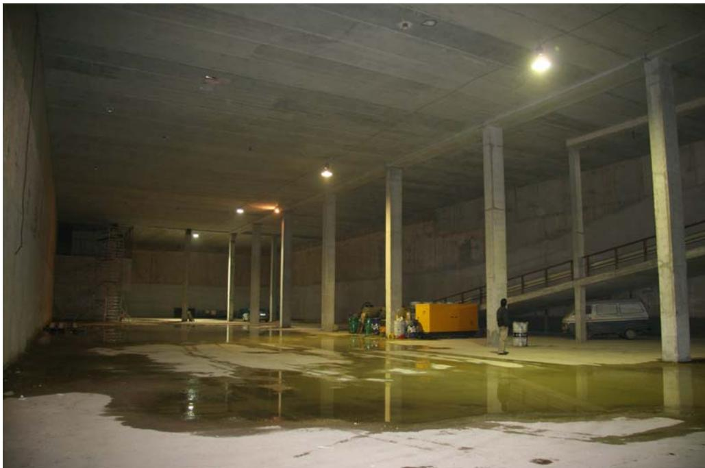
**Fig. 7: Interior view of the 17 x 55 m (56 x 180 ft) column-free area shown in the structural floor plan in Fig. 6**
