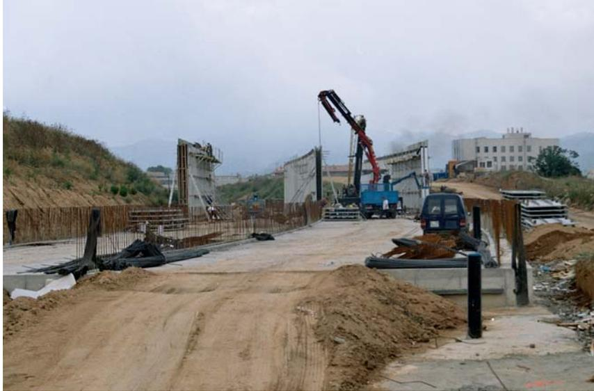
**(a) Semi-prefabricated walls assembly. Note the curvature in plan**
