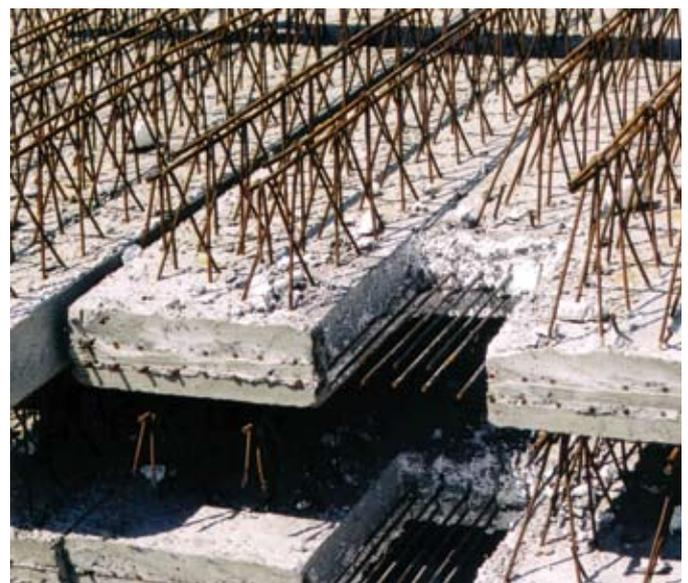
**Fig. 5:** The slab blockout shown here is used in a dropped slab panel spanning between columns and allows the column vertical reinforcement to pass through the precast panel
