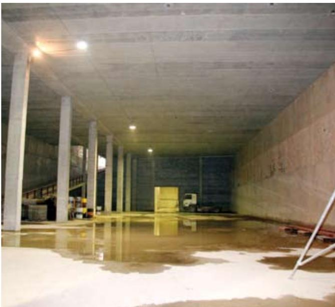
**Fig. 7: Interior view of the 17 x 55 m (56 x 180 ft) column-free area shown in the structural floor plan in Fig. 6**
