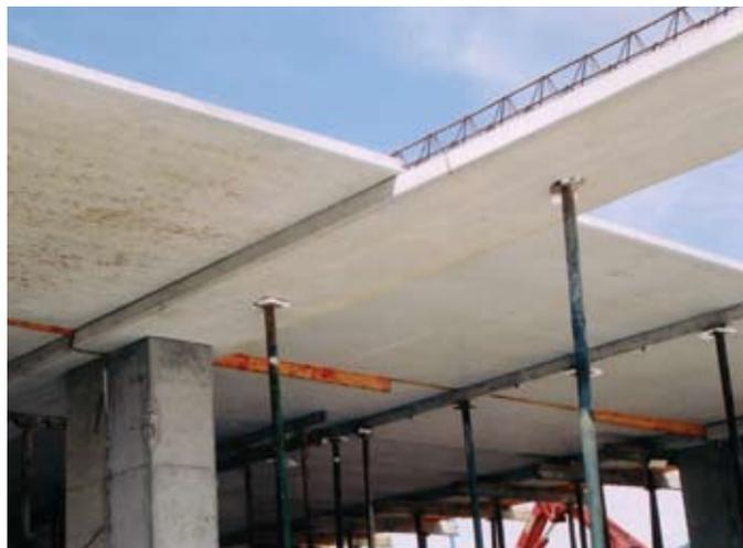
**Fig. 4:** Dropped precast slabs spanning between the columns partially support the precast slabs spanning in the other direction
