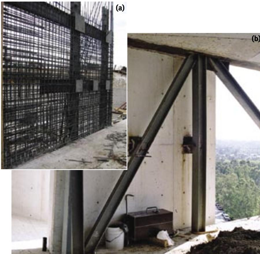
**Fig. 6: Connection between the concrete walls of the central core and the steel trusses supporting the floor plates: (a) during construction; and (b) after installation of the trusses and floor**
