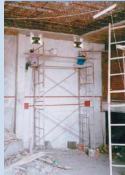
Casino building in Lima, Peru with BOZZO-GERB Dissipators
